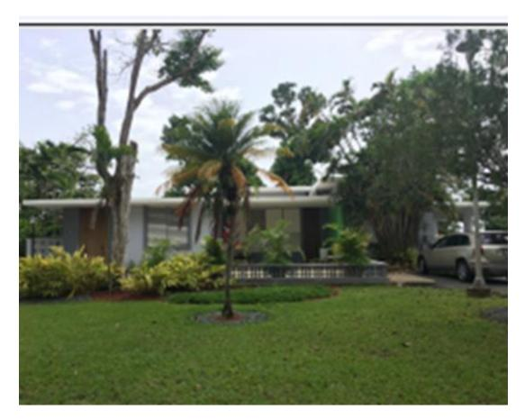
It is a site cast, reinforced concrete building with a reinforced concrete roof with a bituminous built—up roof system. The interior includes reinforced concrete bearing walls with a reinforced concrete floor slab on grade. The facility has an 8FTx10FT attached car port and detached laundry room with bathroom. Interior finishes generally consist of suspended acoustic ceiling, painted concrete or drywall and terrazzo and vinyl floor tile.
