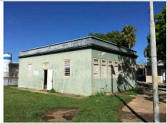
The Baños de Atletas building is a 1,300 SF, single-story bathroom and storage building that was constructed in 1940 (84 years old). The building is a cast-in-place reinforced concrete building with 3-FT parapets on three sides. The roof is sealed with an elastomeric coating. The interior includes reinforced CMU wall partitions. Interior finishes generally consist of plastered ceiling, plastered and painted walls and hydraulic floor tile.
