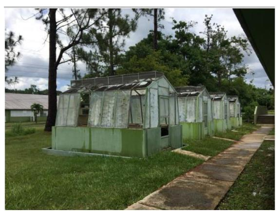
Greenhouses 1, 2, 3, and 4 have a 3-foot reinforced concrete wall supporting a metal frame structure. The roof (225 SF) is made up of glass panels. The interior finishes are made up of glass panels, bird screen, concrete walls and floor. The Greenhouses are located just north of the Entomology Lab.
